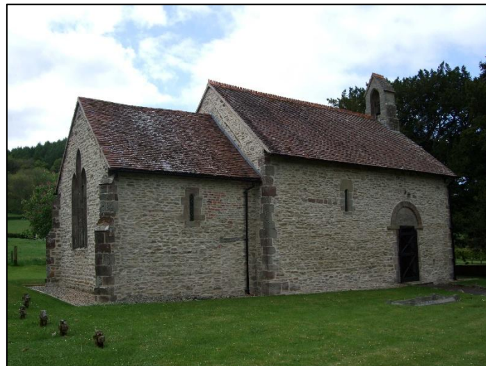
Pipe Aston St Giles
